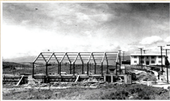
Construction well underway in early 1950
