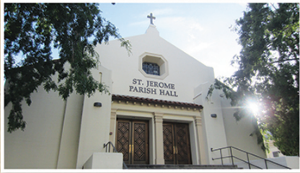
Today our "first" church is now the Parish Hall
